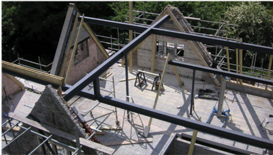
"Structural Steel Work for Residential renovations, Siston, Bristol"
